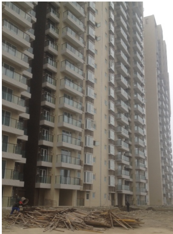
Chengdu Jinniu District Yujia New Homes Project. Feb 20, 2014. Photo by J
