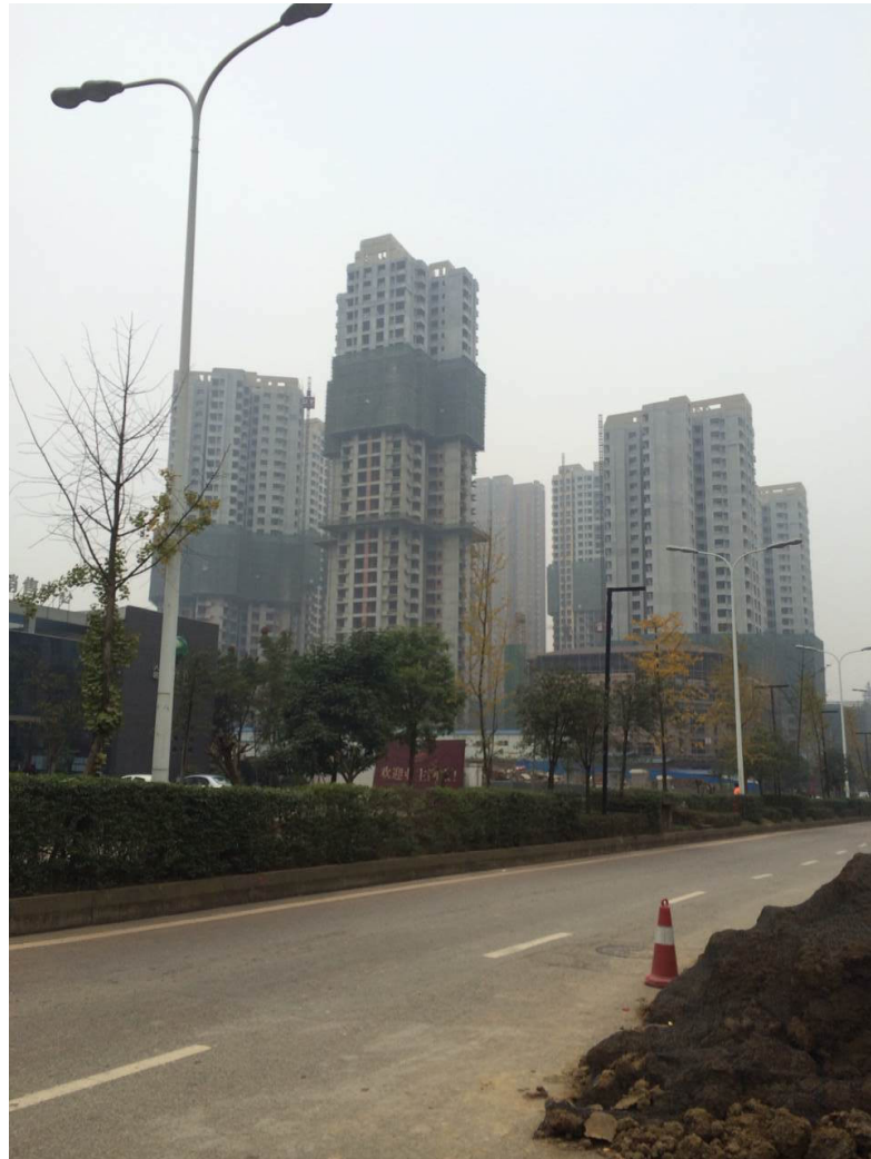
The “468” project under construction. | Photo by J Capital
