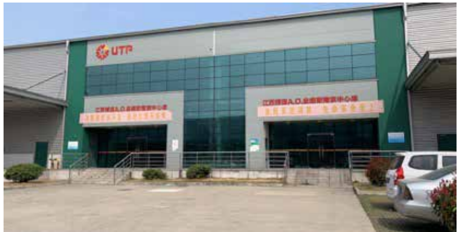
This photograph shows warehouse space owned by UTP and dedicated to AOS. Photo by J Capital March 2019.
