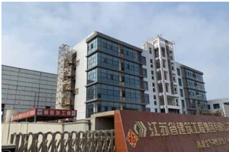
UTP environmental equipment base. Photos by J Capital March 2019.
