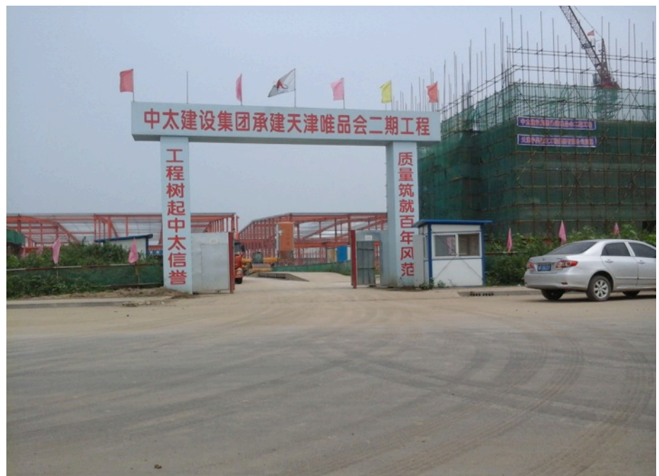
J Capital Research: New Tianjin Warehouse under construction; Aug. 2014
