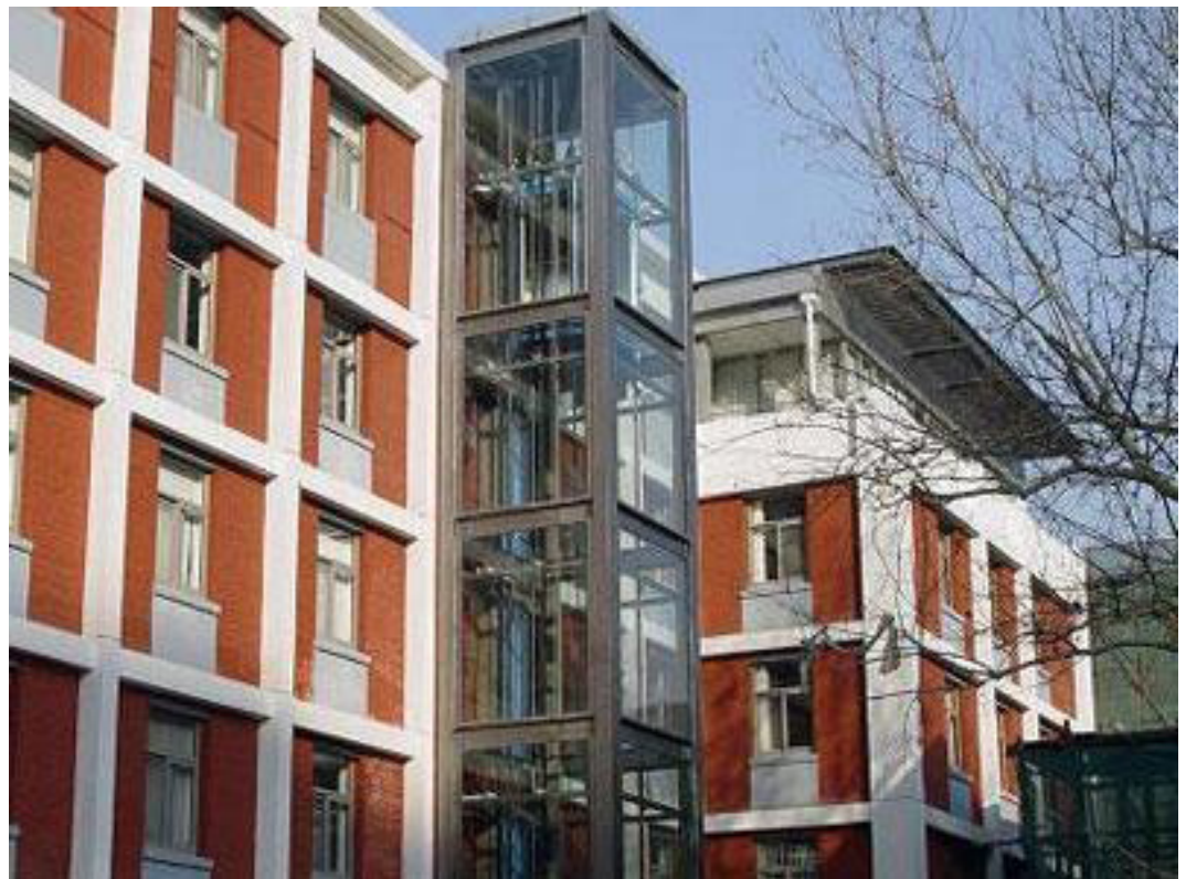
Demand to retrofit external elevators to buildings under seven stories is now a key driver of elevator demand. Source: fang.com
