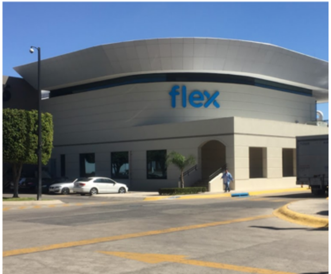
Enphase contract manufacturing facility operated by Flex in Guadalajara, Mexico Source: Google
