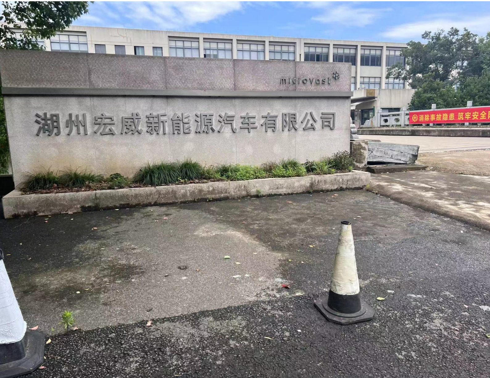
Our photos of the three sites in China show no construction activity and no visible manufacturing. Photos were taken at 3 pm on a Monday.
